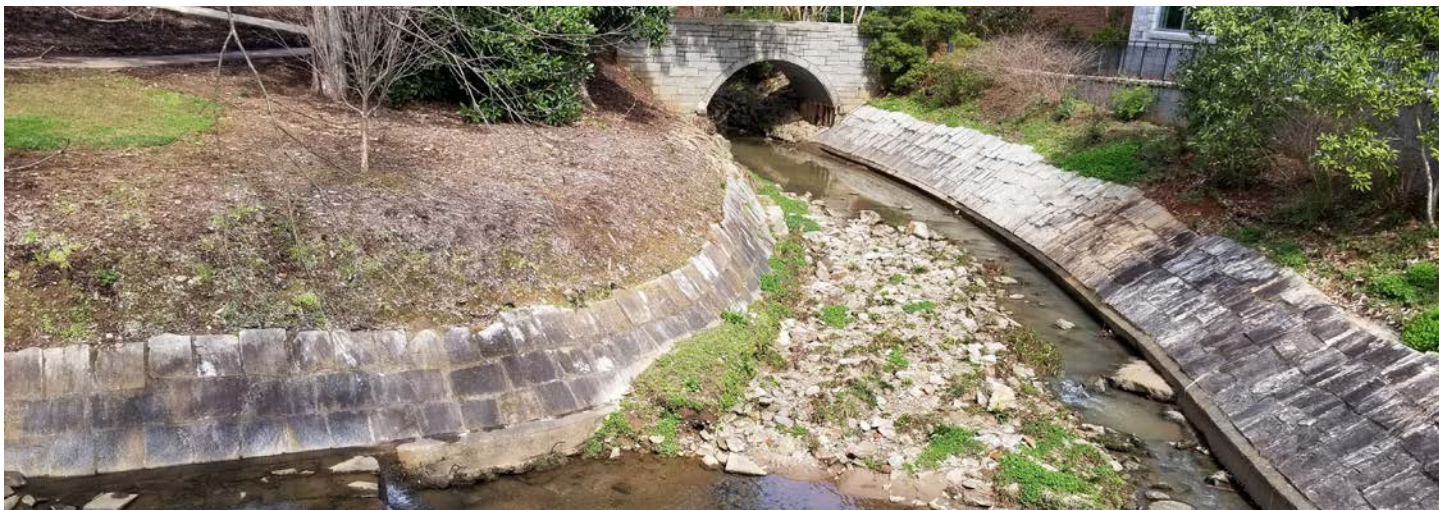
Tanyard branch is channelized for the majority of the reach resulting in similarity to a stormwater pipe.
